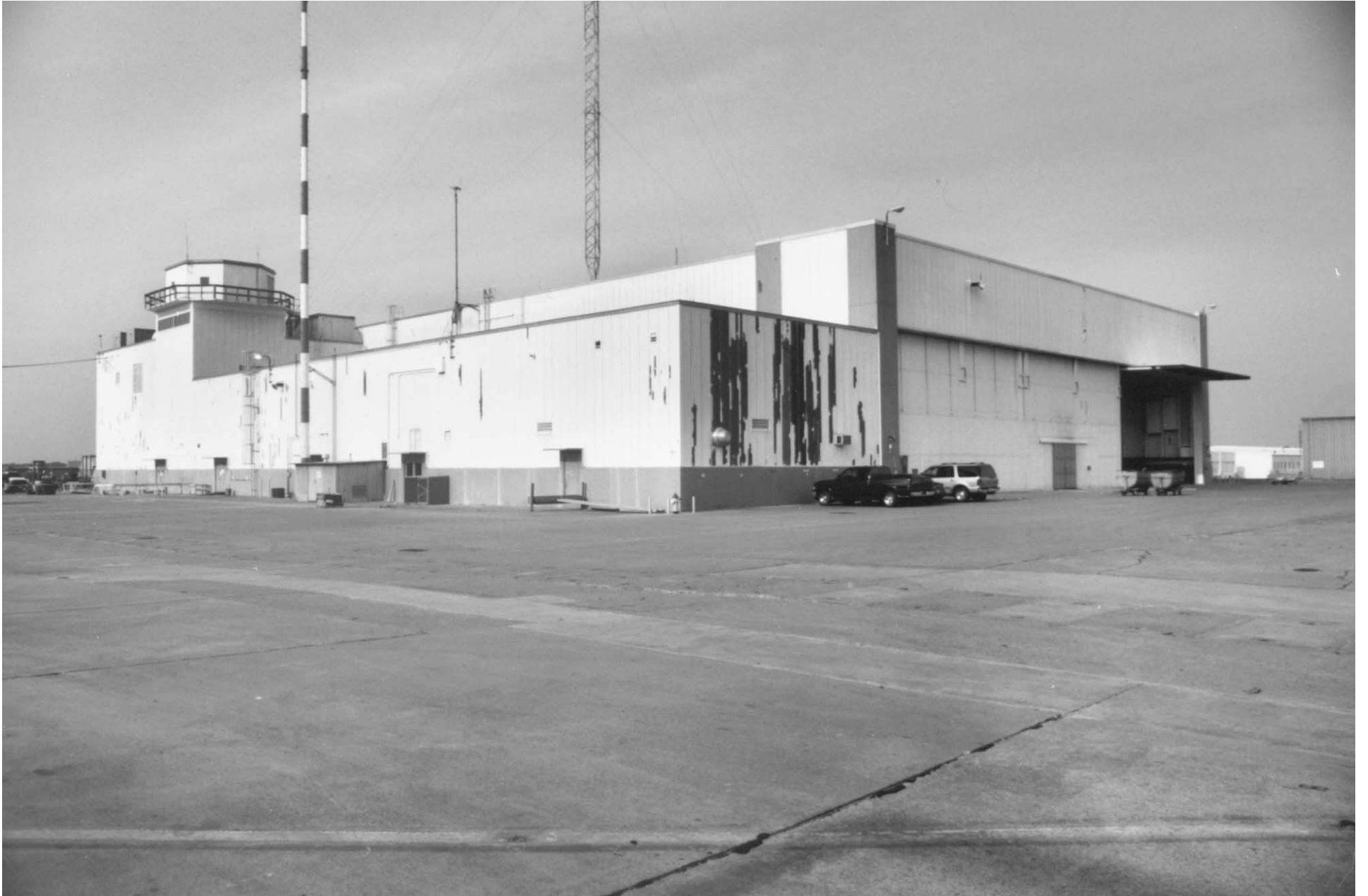
N and E facades of Facility 97, camera facing SW
