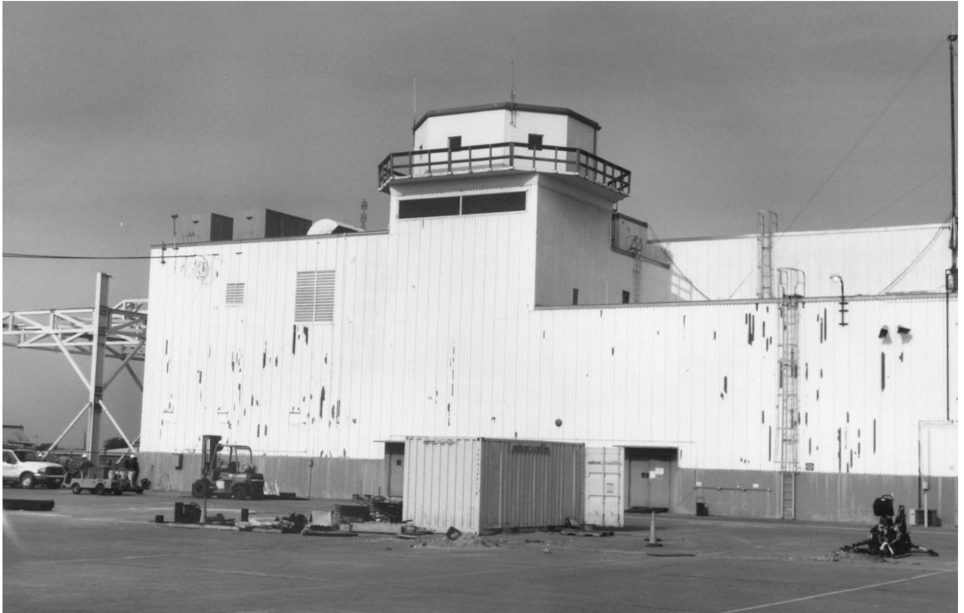
Detail of E facade of Facility 97, camera facing SW
