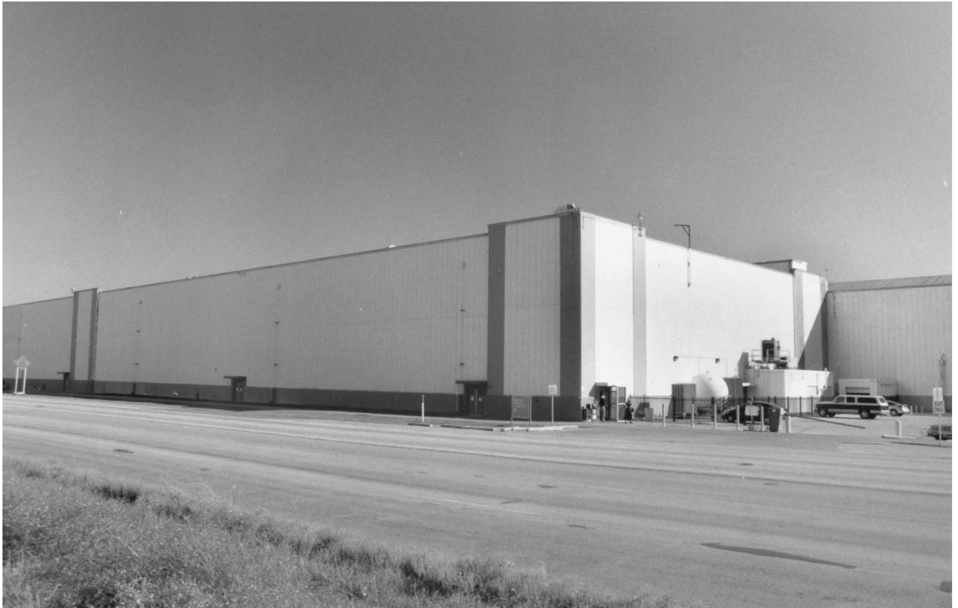
N and W facades of Facility 49, camera facing SE
