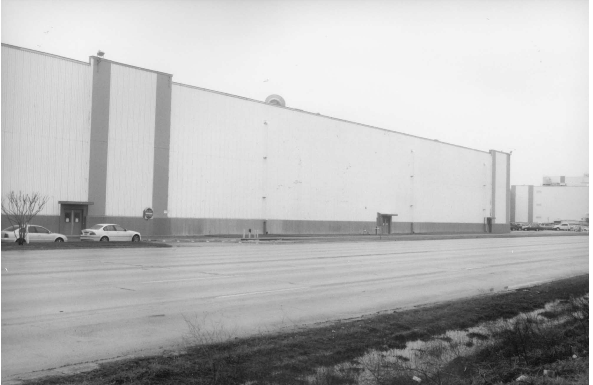
Oblique view of N facade of Facility 49, camera facing SW
