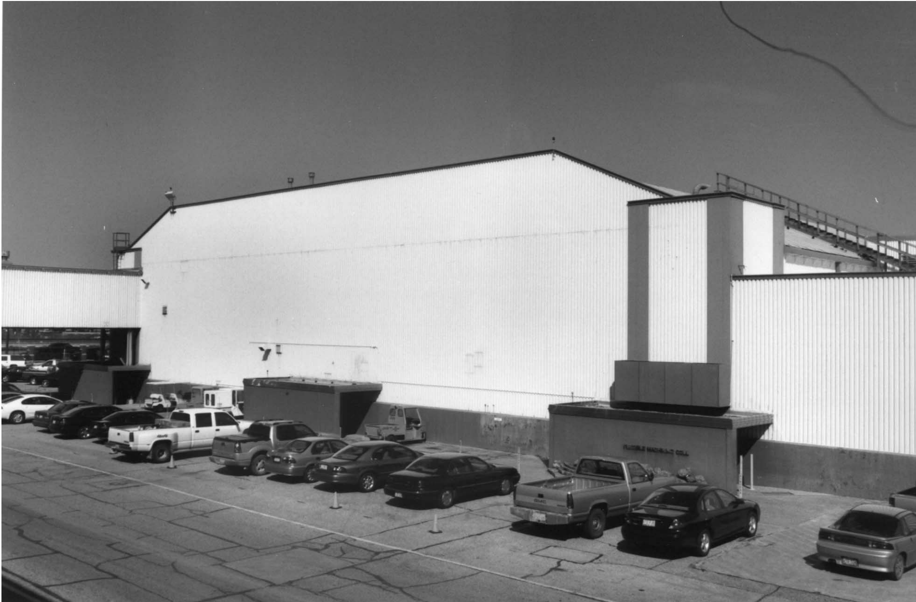
Detail of W facade of Facility 1, camera facing NE
