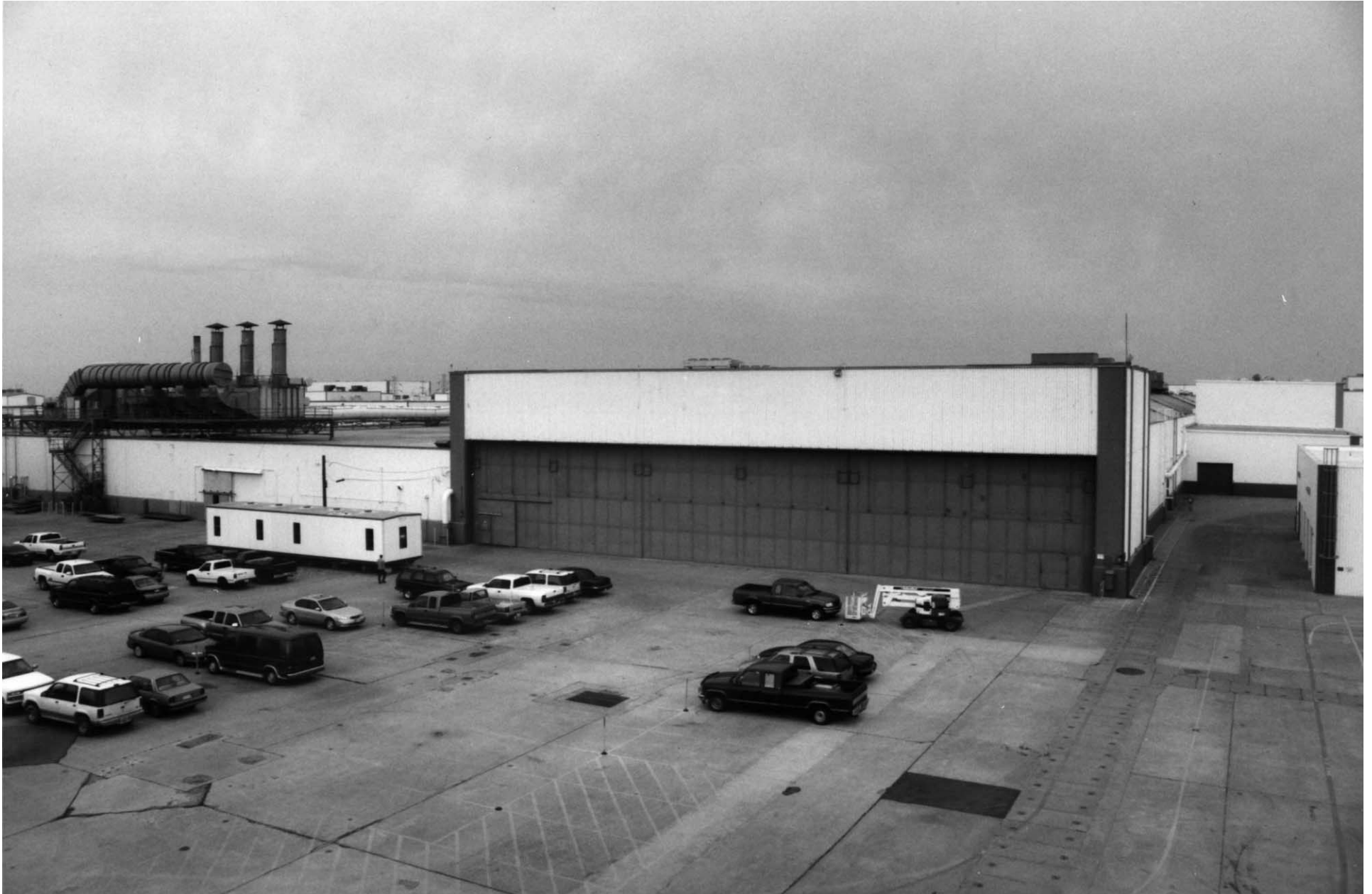
Detail of E facade of Facility 1, camera facing SW
