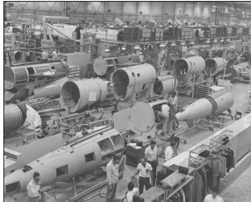
Figure 8-54. Production of the Regulus II.
