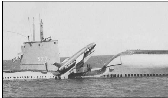
Figure 8-64. Regulus-launching mechanism on the U.S.S. Growler.
