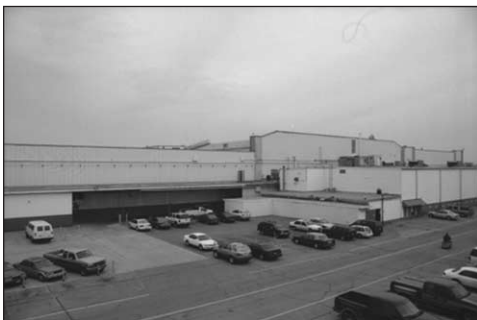
Figure 13-18. Large expanses of flat roofs with raised, gambrel roofs over final assembly areas are characteristic of Facilities 1 and 6 at NWIRP Dallas.
