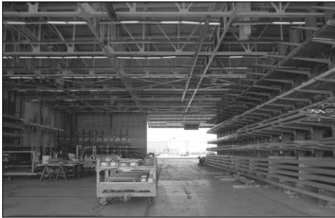
Figure 13-22. The open plan and exposed structure of Facility 97 — which are also characteristics of Facilities 1, 6, 16, and 94 — are important features that should be retained.
