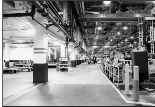
Figure 13-21. Concrete columns, large open spaces, and exposed steel roof trusses are important character-defining features of Facility 6.
